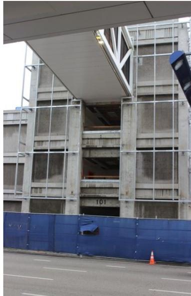
**Elevators are being replaced and metal panels installed at the East tower of PS-1.**
