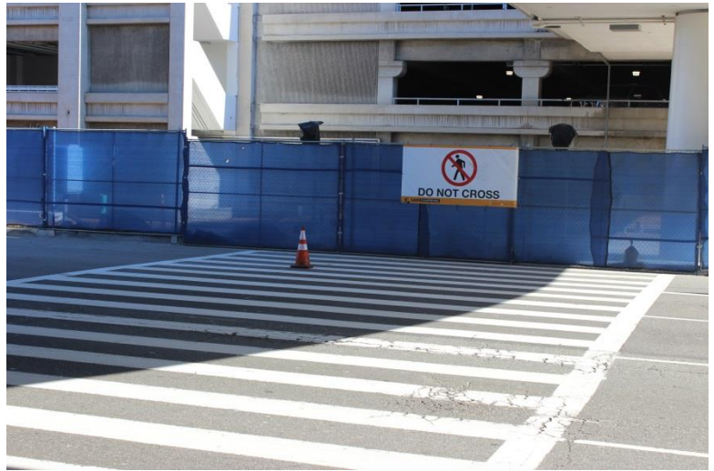
The crosswalk between the Tom Bradley International Terminal and Parking Structure 3 is temporarily closed.
