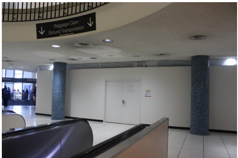
Concessions are being installed in two locations in Terminal 3.
